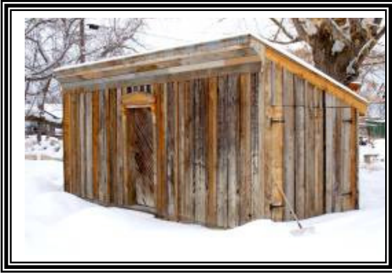
Old shed/new shed: The only thing the Kimball's added to rehabilitate this collapsing shed was new rafters and a door from the even older original barn from which the wood for the original construction was donated.
