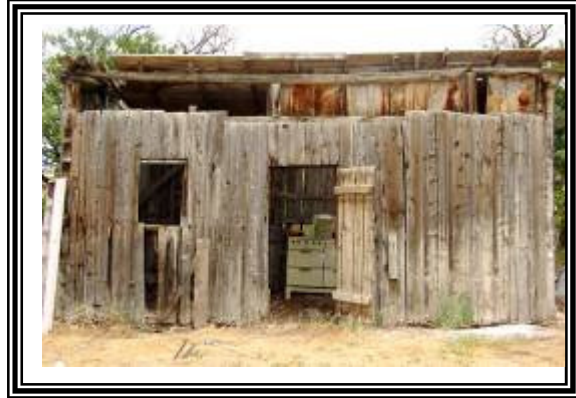
Old shed/new shed: The only thing the Kimball's added to rehabilitate this collapsing shed was new rafters and a door from the even older original barn from which the wood for the original construction was donated.
